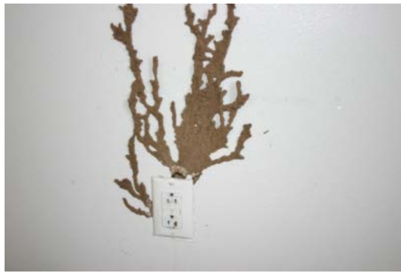
Subterranean termite shelter tubes.
