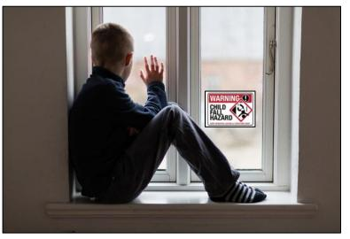
PPV Partners & MHOs have installed safety measures to windows with sill heights of <u>24</u> <u>inches or lower</u> in homes. Windows with sill heights higher than 24 inches may not have secondary safety devices
